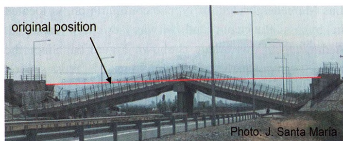
Figure 7: Collapse of Los Pinos underpass, South access to Santiago.
