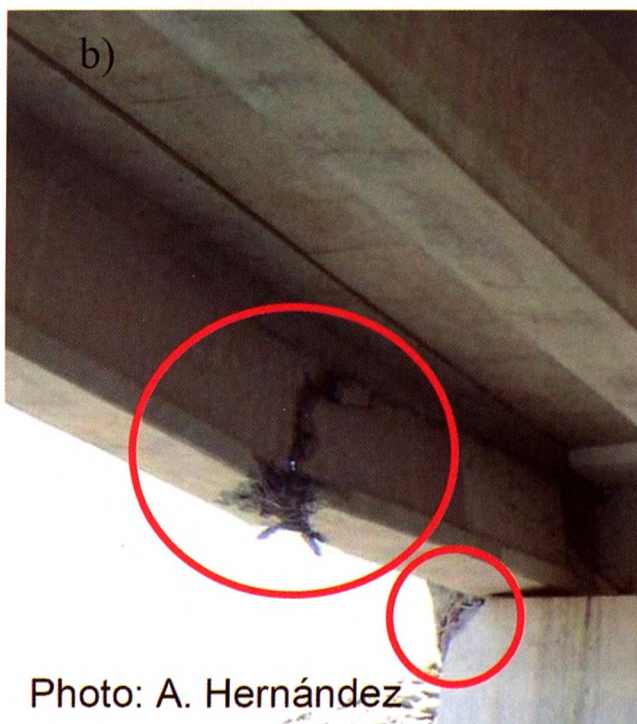
Figure 5: Damage in girders of type 2 bridge configuration, underpass Chada, South access to Santiago.
