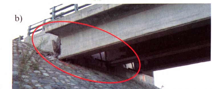
Figure 6: Damage in Las Mercedes underpass, bypass Rancagua, route 5.
