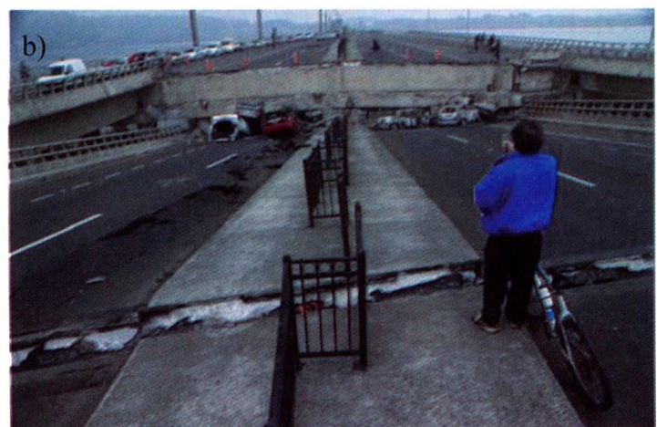
Figure 10: a) Abutment settlement and lateral displacement in Concepción railway bridge and b) collapse in the access to the Llacolén bridge in the Concepción side
