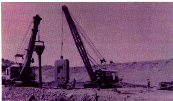
Figure 2: Construction of the slurry wall (Bachy, around 1974)
