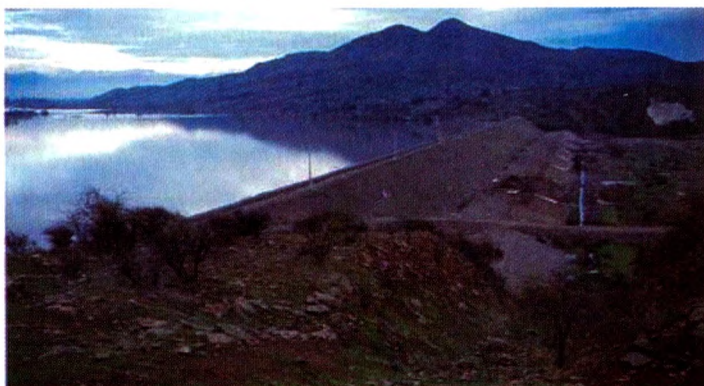
Figure 1: Convento Viejo dam operating only with the cofferdam (ICOLD, 1996)
