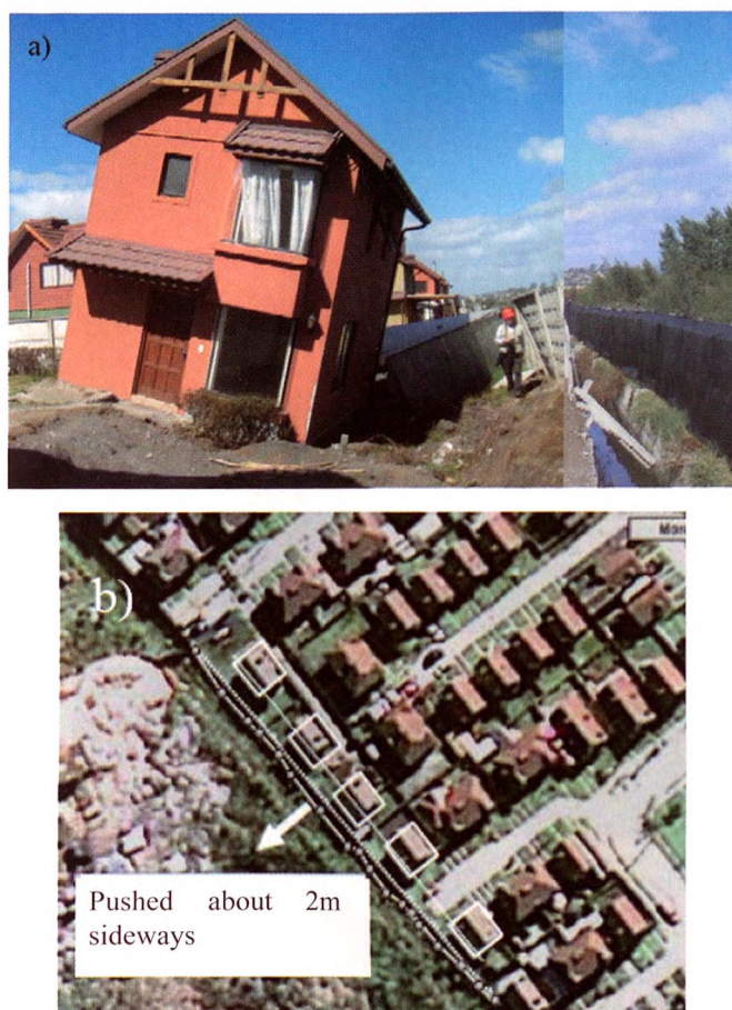
Figure 5: Houses at Brisa del Sol a) significantly tilted house and b) line of houses affected by ground lateral displacement
