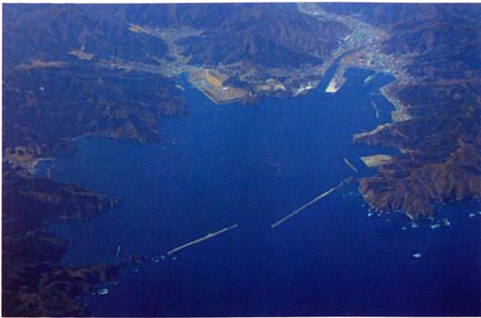
Figure 2: Kamaishi port breakwater, taken from http://www.city.kamaishi.iwate.jp
