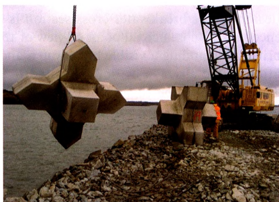
Fig. 7 Installation of Xblocs over a breakwater
