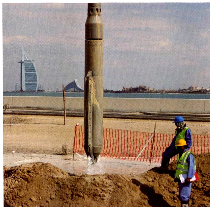
Figure 5: Vibro compaction - Palm Island, Dubai
