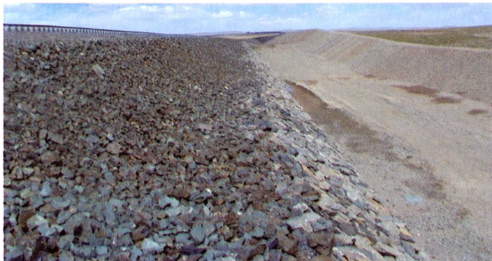
Figure 1: In situ experimental railway section with crushed rock slope protection
