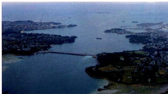
Figure 3: La Rance tidal barrage, France, capacity of 240 MW
